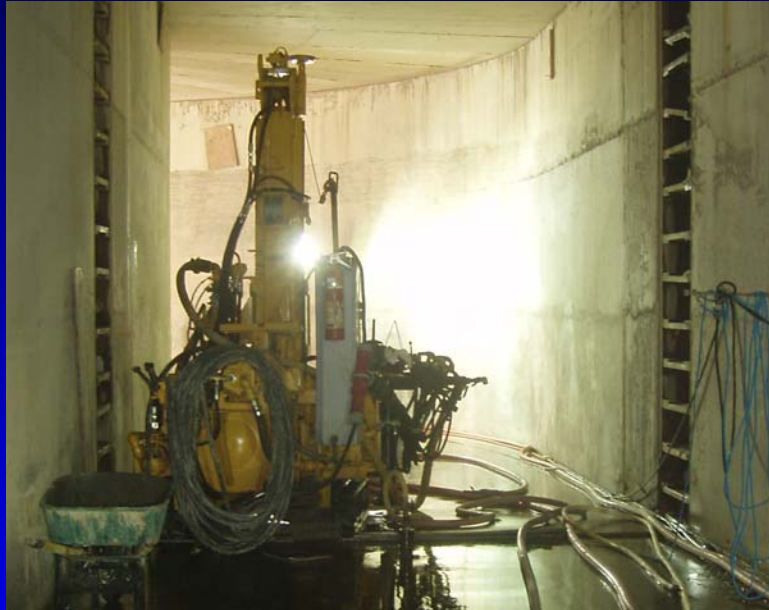
Drilling Grout Holes
