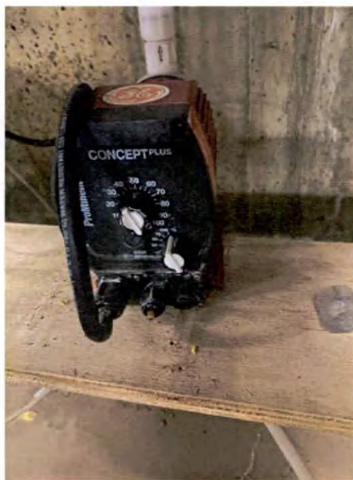
Fine Arts 6 chemical pump 1 close up Fine Arts 7 chemical pump 2
