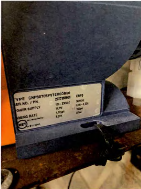
Drinko 4 chemical pump 1 close up
